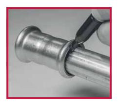
4. Rotate the tube and fully locate tube into the fitting and mark as shown for reference.
